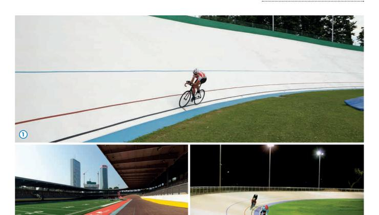
MAPECOAT TNS CYCLE TRACK is a multilayer acrylic resin-based waterborne system designed for velodromes installations. Suitable for indoor and outdoor installations, both on concrete and asphalt substrates. MAPECOAT TNS CYCLE TRACK, thanks to the high wear resistance, offers an excellent combination of sliding properties and stability for the athlete during the sport performance.
