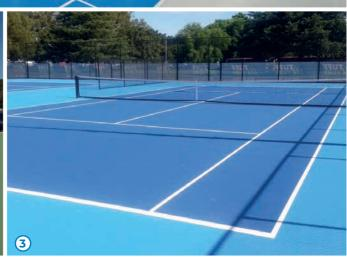
MAPECOAT TNS CUSHION is a multilayer semi-flexible acrylic resin-based waterborne system designed for prograde tennis courts installation. Suitable for indoor and outdoor installations, both on concrete and asphalt substrates. Forms a highly resistant, even playing surface for safe, high-speed rallies with consistent ball bounce. ITF 3 certified system.
