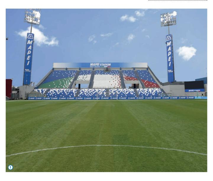
MAPECOAT TNS ARENA WP is a multilayer system, in combination with PURTOP polyurea systems, used for the waterproofing and protection of concrete in stadiums grandstands and/or high footfall area in sport facilities. The high mechanical resistance of PURTOP waterproofing membrane, combined with the anti-slippery properties of MAPECOAT TNS ARENA WP coloured protective top coating, increase both the durability and safety of the sport facility.
