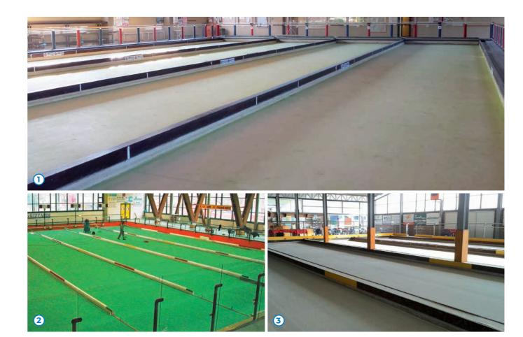
PU PROFESSIONAL is a multilayer polyurethane resin-based system used to create sports surfaces for playing bowls. Suitable for indoor and outdoor installations, both on concrete and asphalt substrates. High resistance to impact loads from bowls balls, with a finish to promote precision bowling and guarantee high performance surfaces that resist wear over the years.
