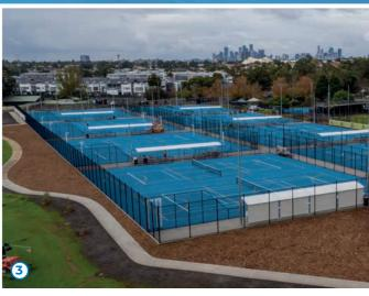
MAPECOAT TNS PROFESSIONAL is a multilayer acrylic resin-based waterborne system designed for prograde tennis courts. Suitable for indoor and outdoor installations, both on concrete and asphalt substrates. Forms a highly resistant, even playing surface for safe, high-speed rallies with consistent horizontal ball bounce. ITF 1 certified system.
